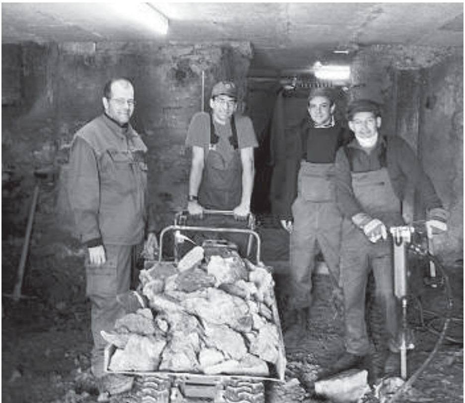
Arbeiten in Eggerberg VS.
